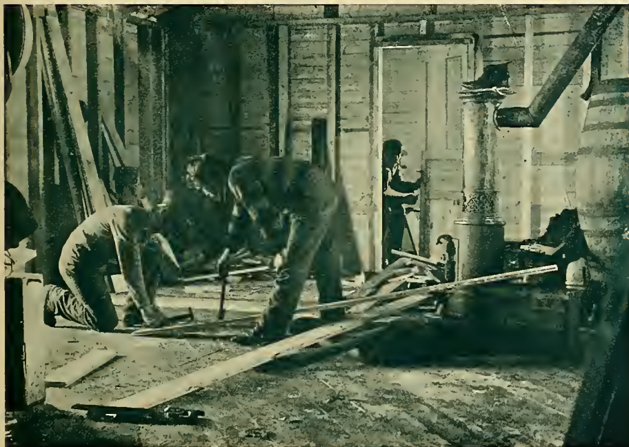
LAYING THE FLOOR
